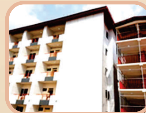
Medical Ward Extension - Laje , Ondo
