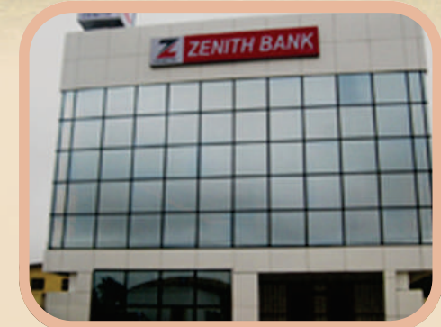
Building COstruction - Zenith Bank
