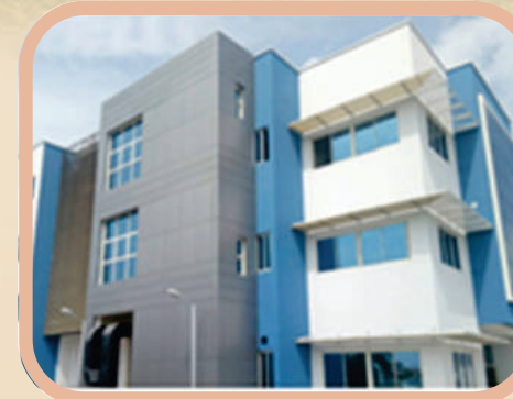
Construction of Studio- Channel TV
